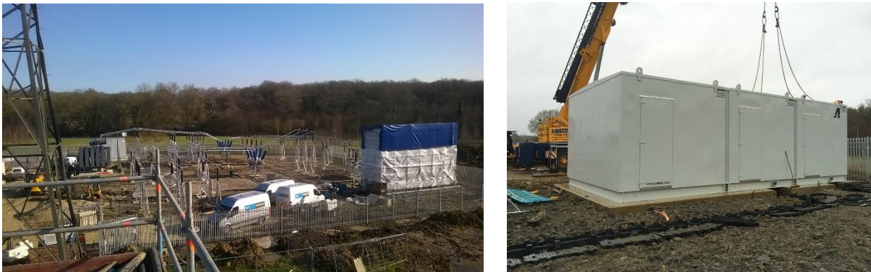
Figure NTS-10: Substation compound under construction
