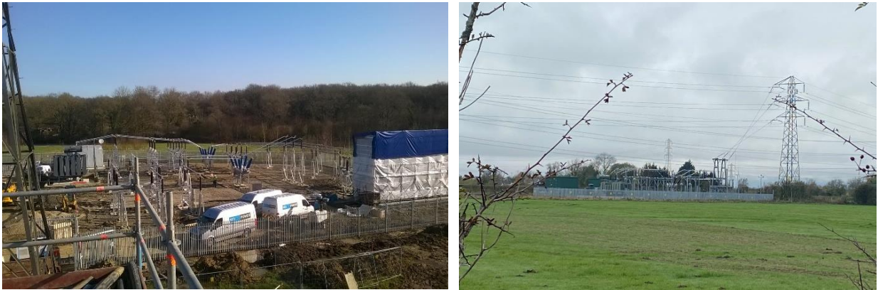
Figure 2-11: Substation compound under construction (left) and completed substation compound (right)
